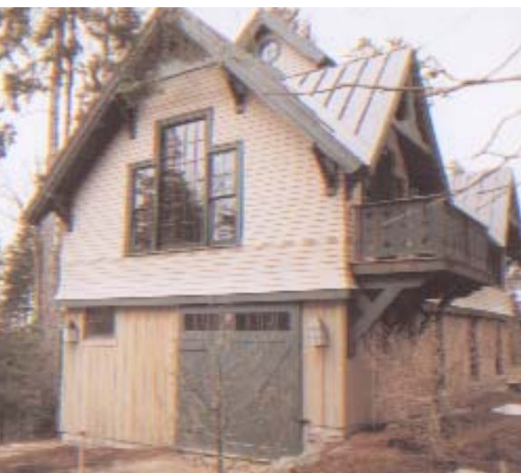
Exterior finishes diminish an imposing structure. Board-and-batten western red cedar covers the first floor; eastern white-cedar shingles cover the second floor. Photo taken at C on floor plan.
